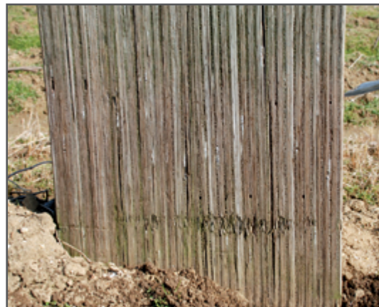
Pole foot with soil foundation after 20 years of installation
